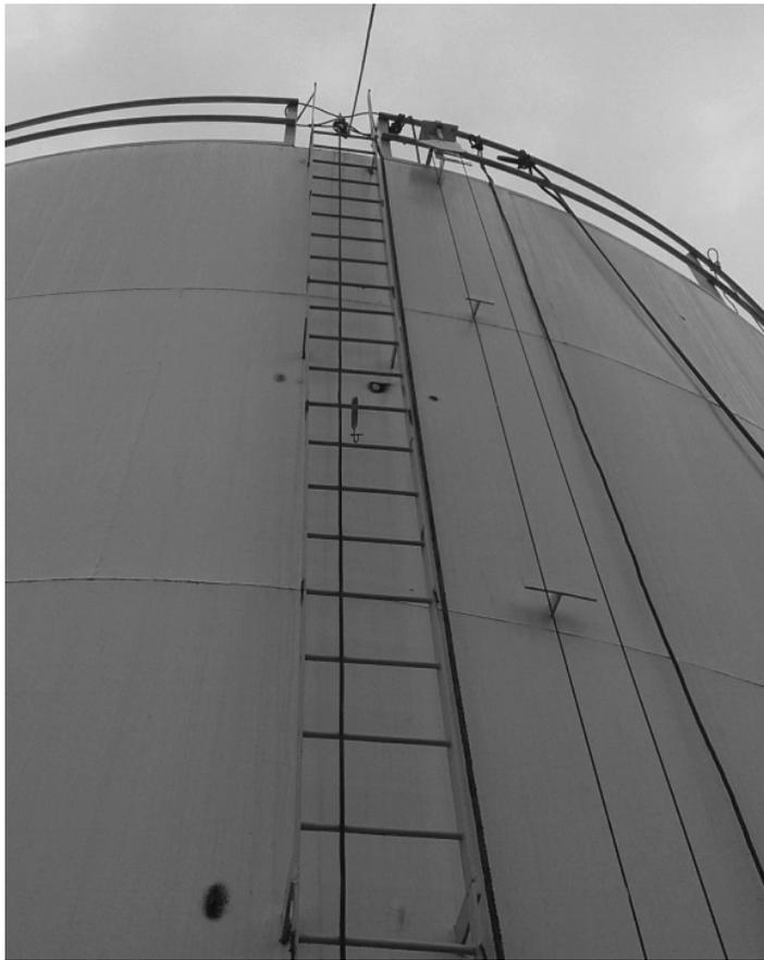
is connected to the cable and the slide is hooked onto a climber's harness. Ladder guards prevent intruders from easily accessing the tank. Round ladder rungs don't offer an edge or grip of any kind, but anti-skid rungs do. They must also be at least 16" wide and should have anti-skid rungs to prevent slips and trips.
