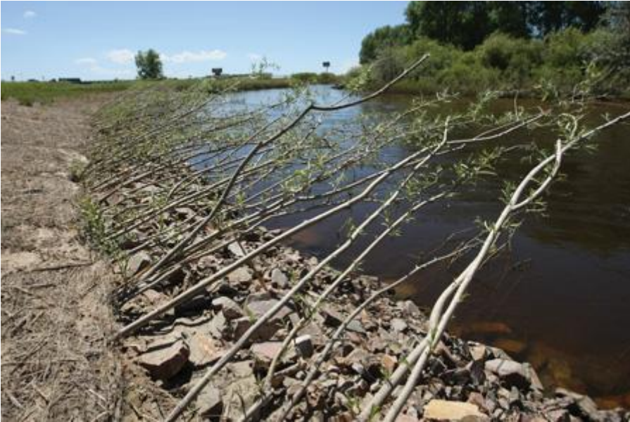
Willow trees planted by the Laramie Beautification Committee help prevent erosion along the Laramie River. Andy Carpenean/Boomerang photographer
