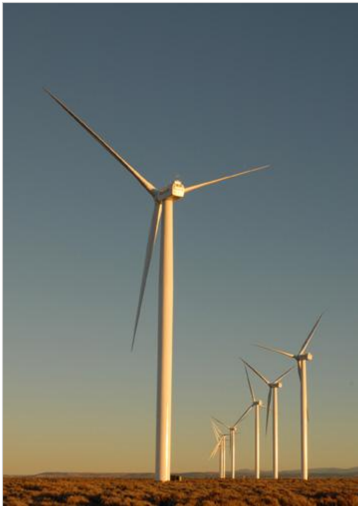
Wind turbines operate in eastern Uinta County. The company that constructed this wind farm also plans to place up to 237 turbines near Rock Springs in adjacent Sweetwater County. (Paul Ng, Star-Tribune correspondent)
