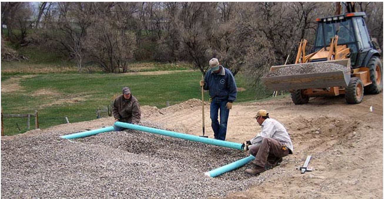
SEPTIC SYSTEM COMPLETED WITH GRANT MONEY: One of 45 septic system clean-up projects completed by Washakie County Conservation District was at the Gene Schreibeis home south of Worland. Above, the new septic tank is lowered into the ground; below, the leachfield is installed for the new tank.
