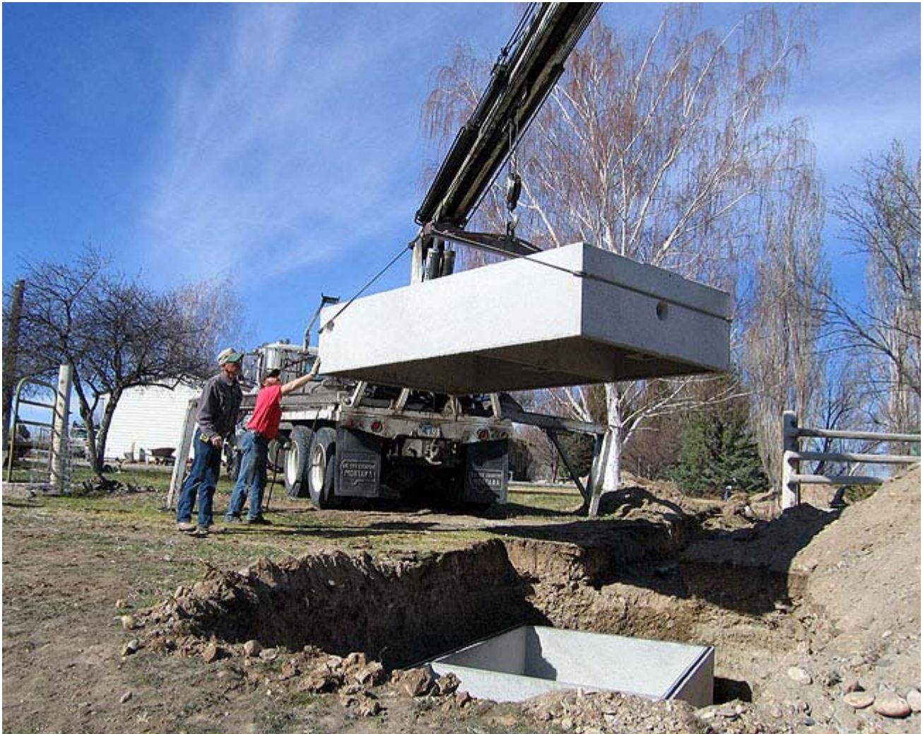
SEPTIC SYSTEM COMPLETED WITH GRANT MONEY: One of 45 septic system clean-up projects completed by Washakie County Conservation District was at the Gene Schreibeis home south of Worland. Above, the new septic tank is lowered into the ground; below, the leachfield is installed for the new tank.
