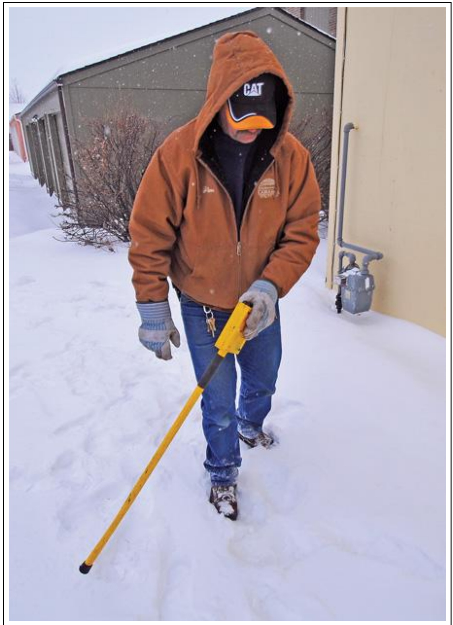
Jim Moody, a utility maintenance operator with the city of Laramie, uses a metal detector to find a water meter underneath the snow Wednesday. Andy Carpenear/Boomerang photographer
