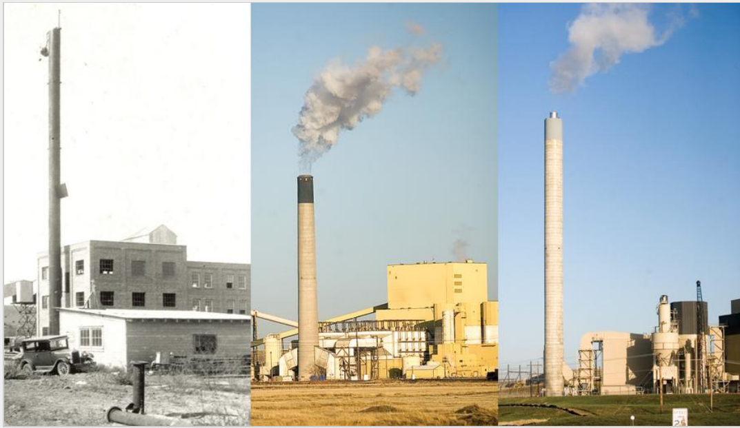
The 1920s-era photo at left shows an original coal-fired steam plant built on the ground where the Neil Simpson I plant was later built. The massive Wyodak plant is in the center. And, at right, the WyGen II plant, completed at the end of 2007, releases a thin stream of steam. — Campbell County Rockpile Museum photo-News-Record photo-News-Record photo by Nathan Payne
