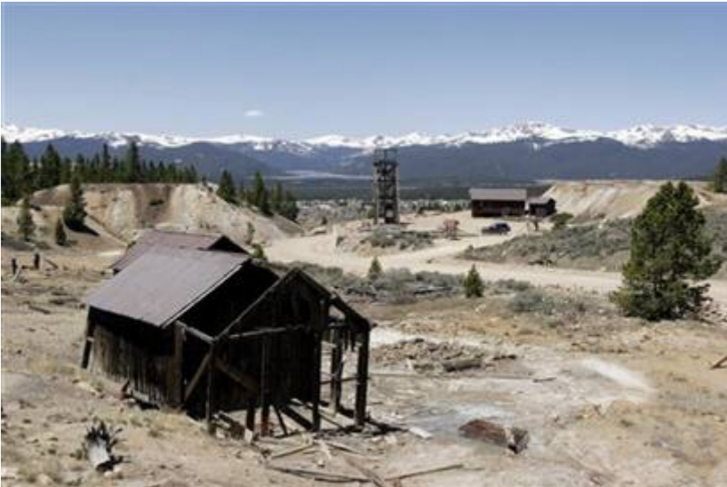
Old mining buildings and shafts east of Leadville, Colo., pictured on Friday, May 27, 2005.
